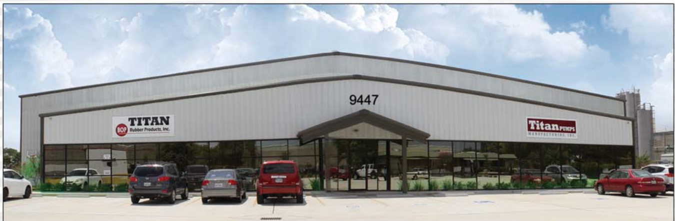
Titan Manufacturing Facility: 45,000 sq. ft.
